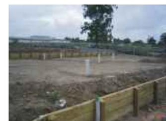
The pipes are left sticking up out of the ground, to stop debris falling down the pipes a cap or tape is placed over the open ends.
